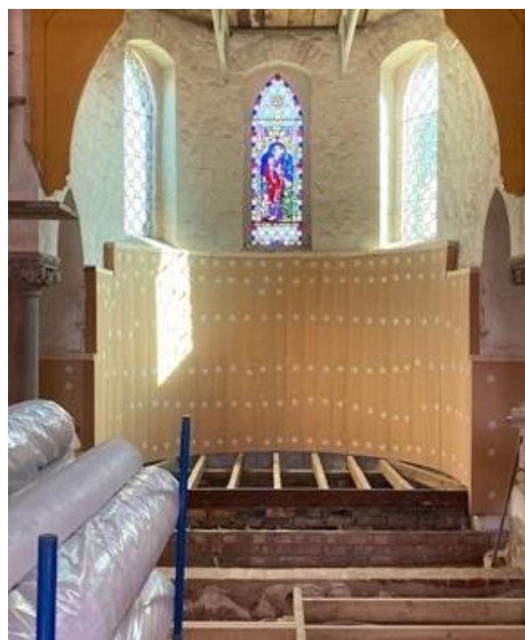
Wall insulation on the lower part of the walls
